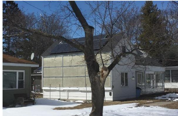
When the panels do not produce enough electricity, the Consumers Power grid supplies the rest. When the panels produce more electricity than he can use, the excess electricity sold back to Consumers Power at the same rate he pays for it. Thus the grid acts as Richard's "storage system" making batteries unnecessary. Consumers Power does charge a minimal monthly fee for this service.
